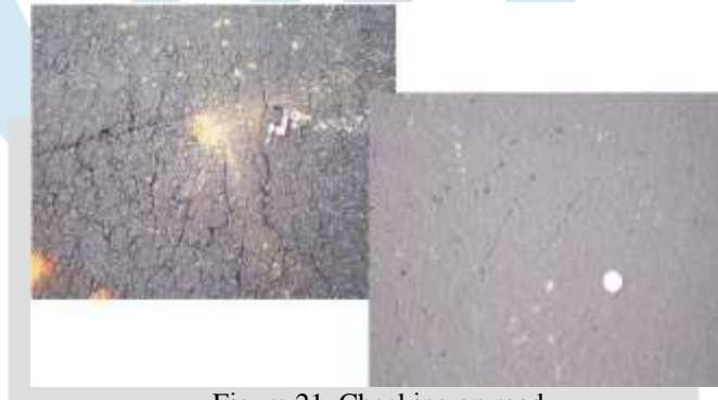
Figure 21. Checking on road
