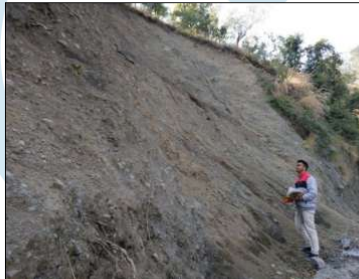
Fig. 3.0 Site View of Salri
