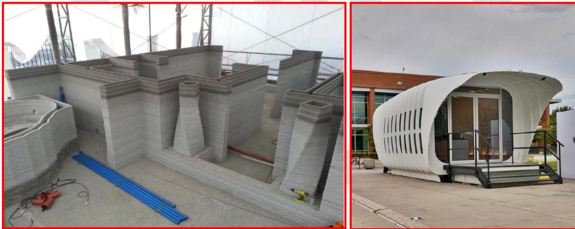
**Fig. 2 Construction of the 3D Printed Villa (Eddie, 2015)**
