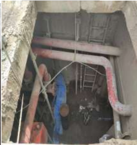
3.RCC Cutout done complicated area
