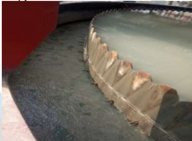
Fig No: 6 Slurry pH 12.5 Clarifier Over Flow : Cationic coagulant Polymer Application
