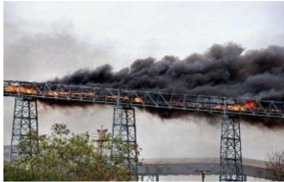
Fig 3 Conveyor belt fire incident
