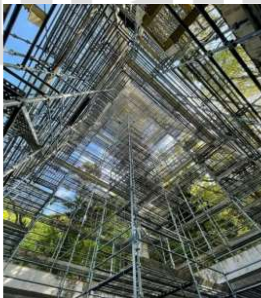
Fig 2 Typical Erection of Scaffold
