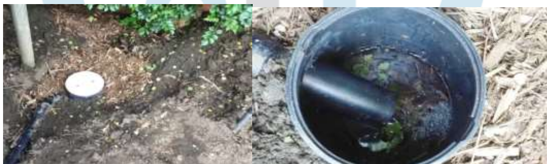
Fig.11: Branch drain grey water System
