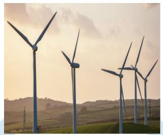
Wind turbines, like windmills, are mounted atop a tower to maximise energy capture. When they reach 100 feet (30 metres) or higher above land, they can take advantage of the faster,
