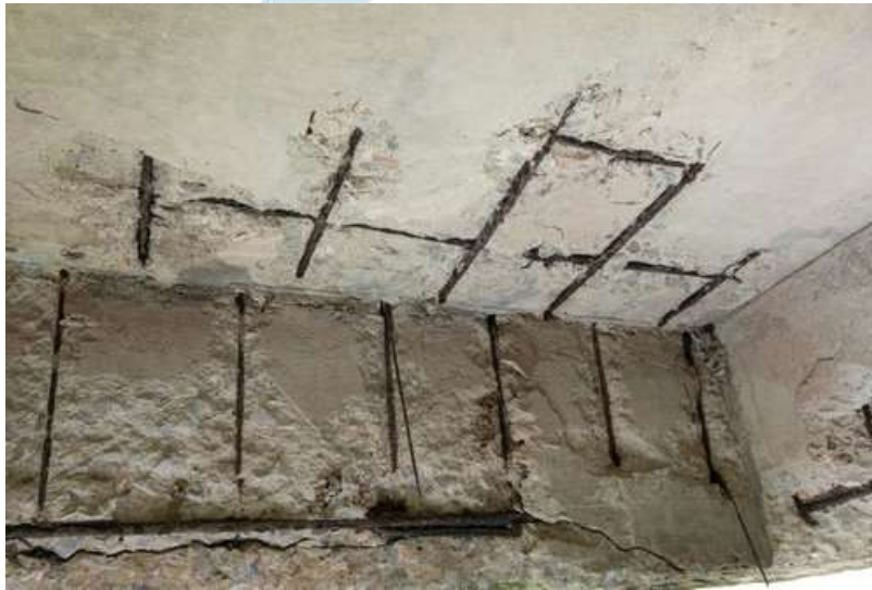
FIGURE 2 : Concrete Spalling and cracking
