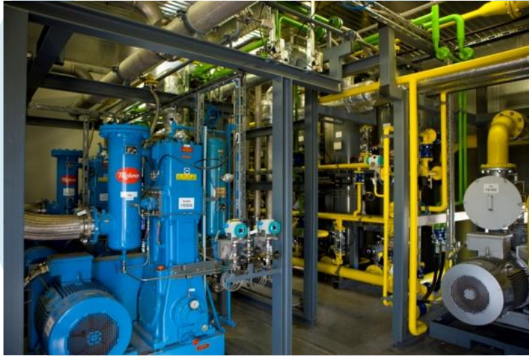
Picture 4: Biogas purification system for CO 2 removal
