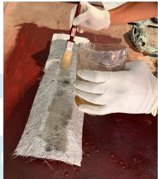
Fig – 27 Glass Fiber Reinforcement Preparation
